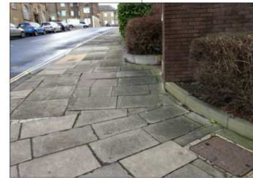
View of corner on Cow Green - several utilities can be seen
