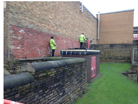
Gas Meter Enclosure
