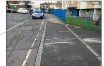
Evidence of gas supply to adjacent property down Swine Market
