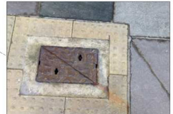
Evidence of water supply valve in Cow Green
